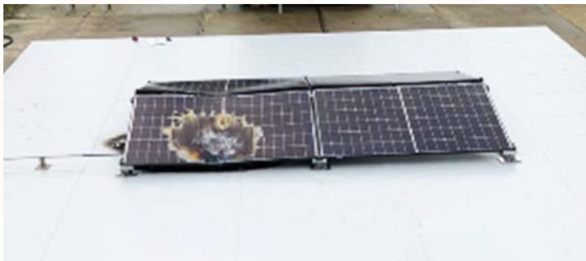
Figure 4: Flat roof with EPS rigid foam and overlying cement-bonded particle board (12 mm here)– damage pattern showing negligible fire spread.
