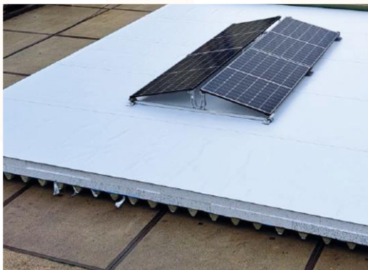
Figure 2: Tested PV system consisting of glass-film modules in an east-west orientation.
